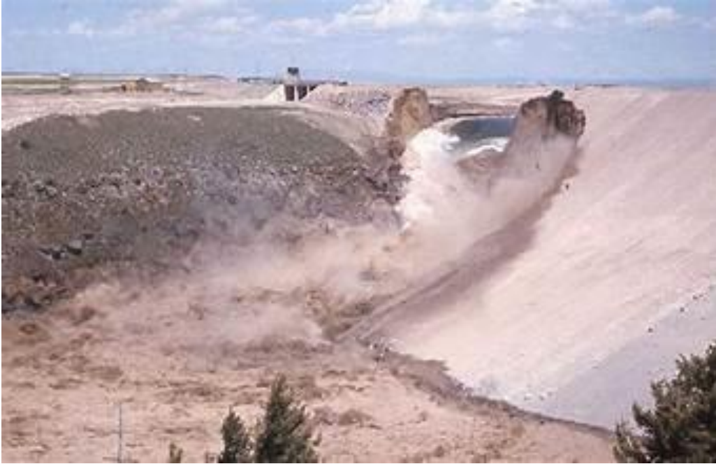
Figure 1:Teton Dam Failure
