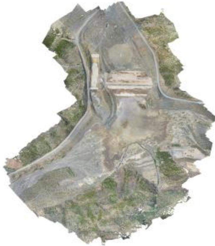
Figure 33: Aerial View of Dam Site
