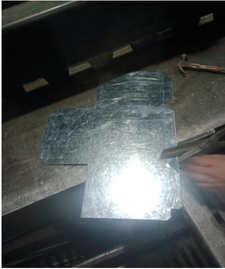
Figure 10 Cutting of sheet
