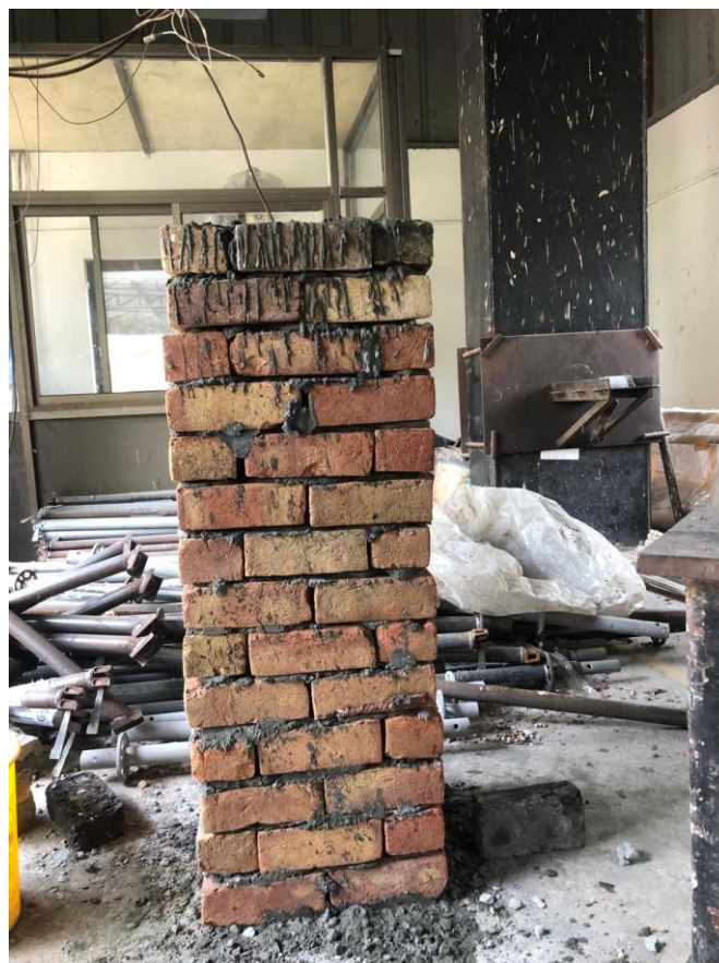
Figure 5: Casting of Column
