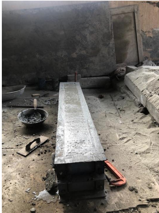
Figure 2: Casting of Beam 2
