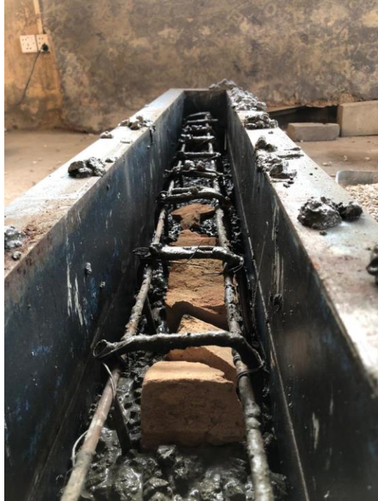
Figure 1: Casting of Beam 1
