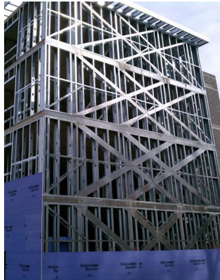
Figure 1.3: Strap Bracing Design
