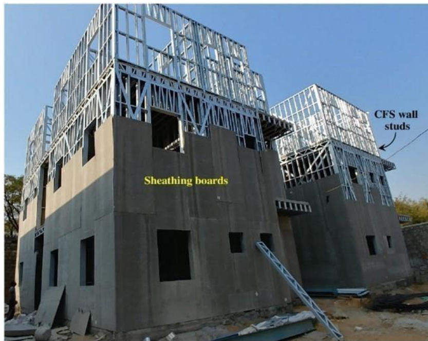
Figure 1.4: Sheathing Brace Design
