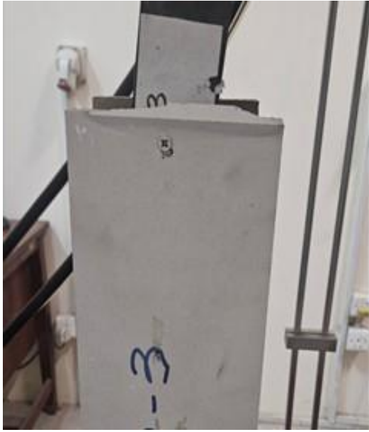
(k) GYP-3 bearing failure/ edge-tearing (B+E)
