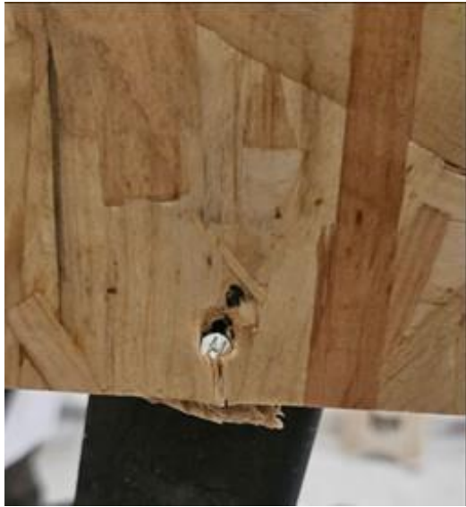
(g) OSB-7 bearing failure/ edge tearing (B+E)
