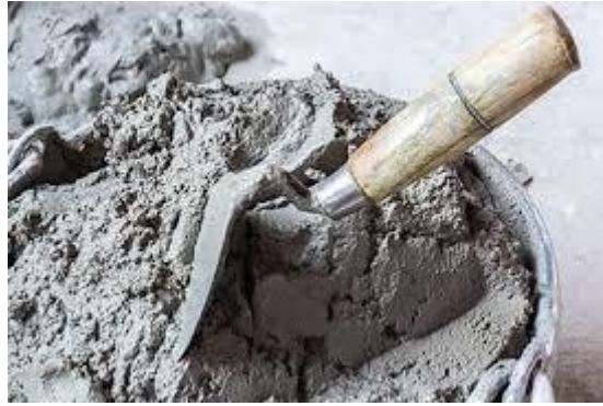
Figure 3.5 Mixing of Mortar
