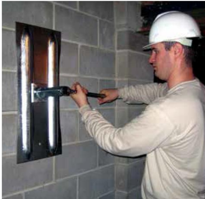
Figure 2.5 Tightening interior wall plate
