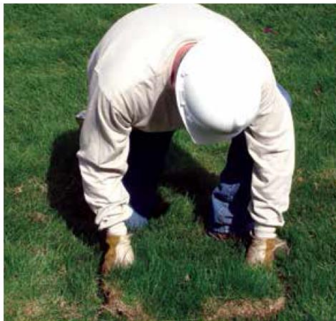
Figure 2.6 covering hole after anchor installation
