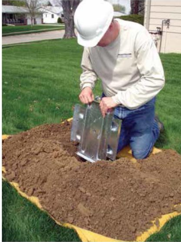
Figure 2.4 Placing exterior wall plate
