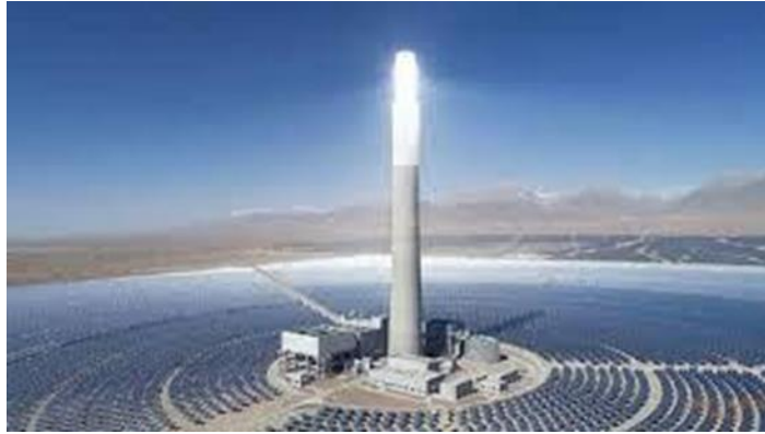
Figure 1.6: 100 MW Concentrated Solar Power Tower project, China [10].
