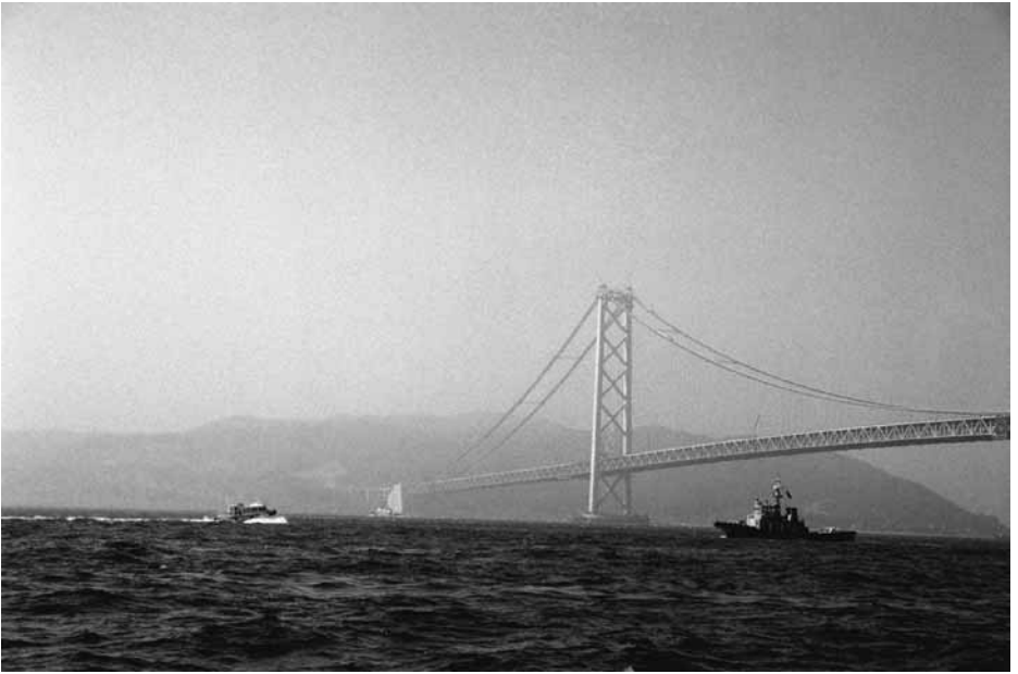
Figure 12.1 Akashi-Kaikyo Bridge, Japan.
