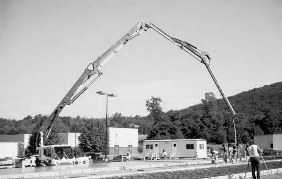
Figure 11.3 A placing boom works well on outdoor pours
