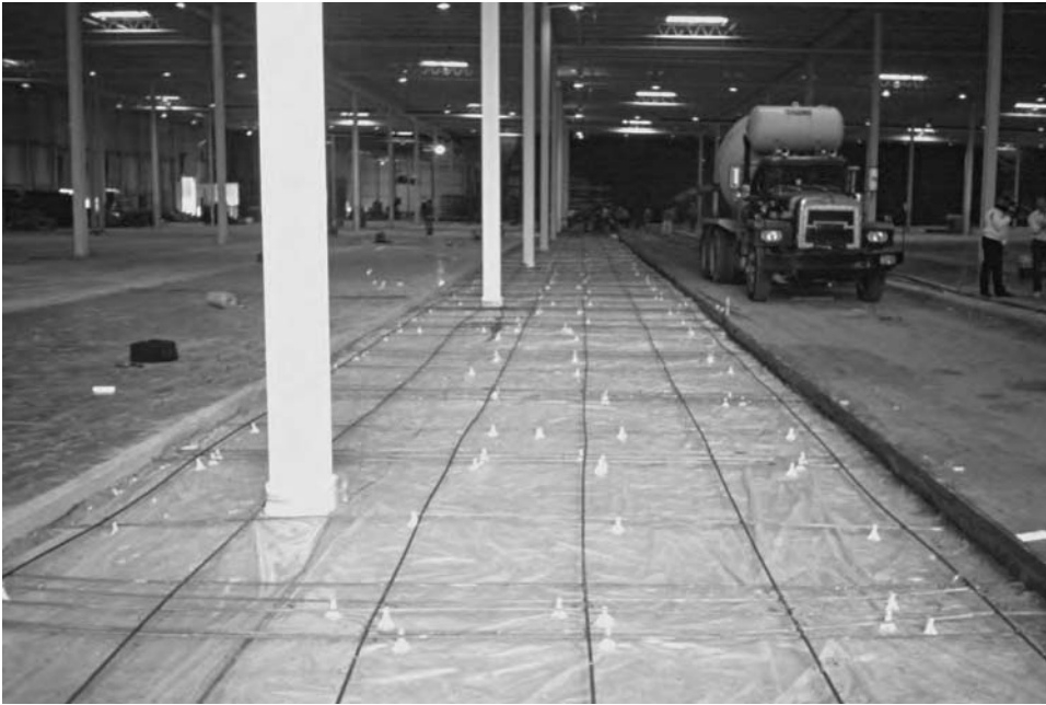
Figure 16.4 One-way post-tensioned floor with unbonded tendons
