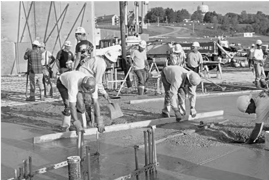
Figure 17.1 A hand straightedge is used for wet screeding
