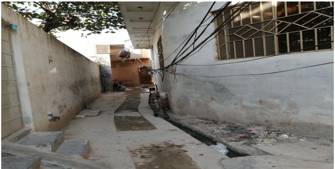
Figure 11: Open Gutters/ Drainage systems in the streets of ghareeb-a-abad
