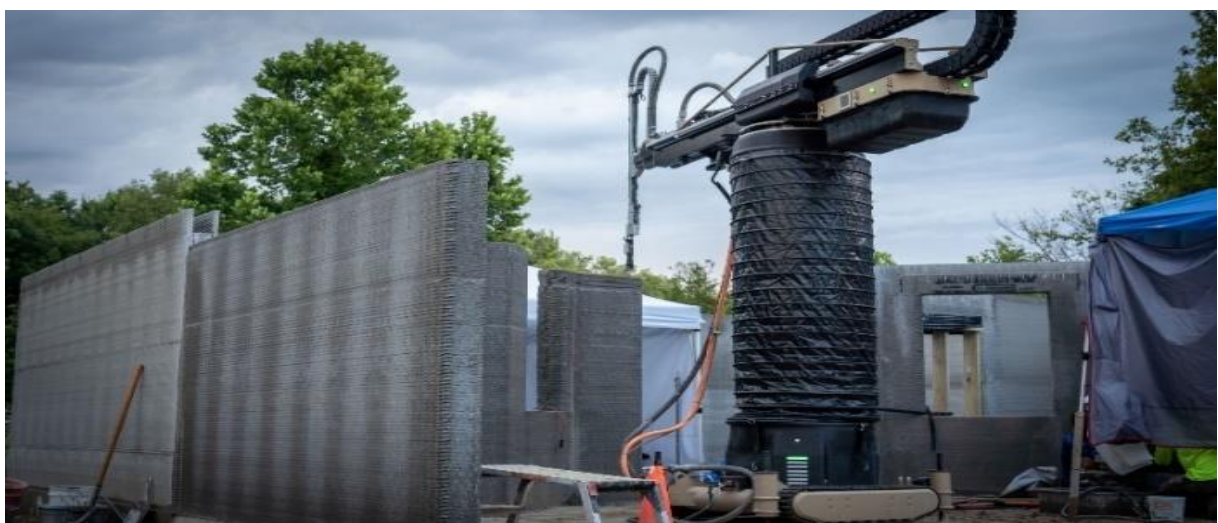
Figure 2-2: 3d concrete printer (Apis Cor, 2019)
