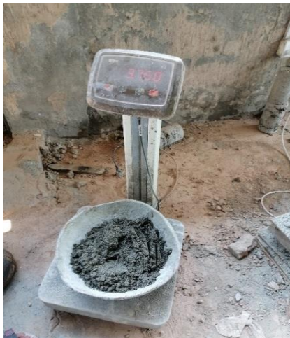
Figure 3-8a Batching Fine Aggregate
