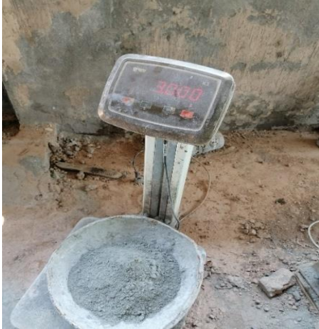
Figure 3-8c Batching of Cement
