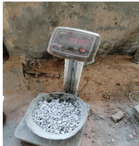
Figure 3-8b Batching Coarse Aggregate
