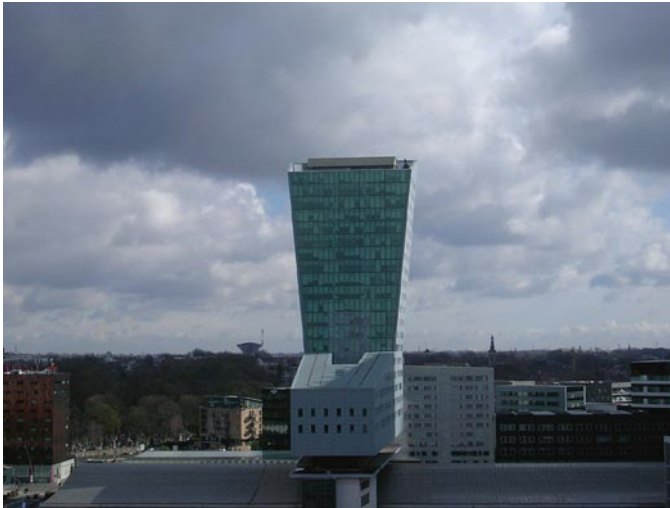
Image 2.4 Building the foundations of security
