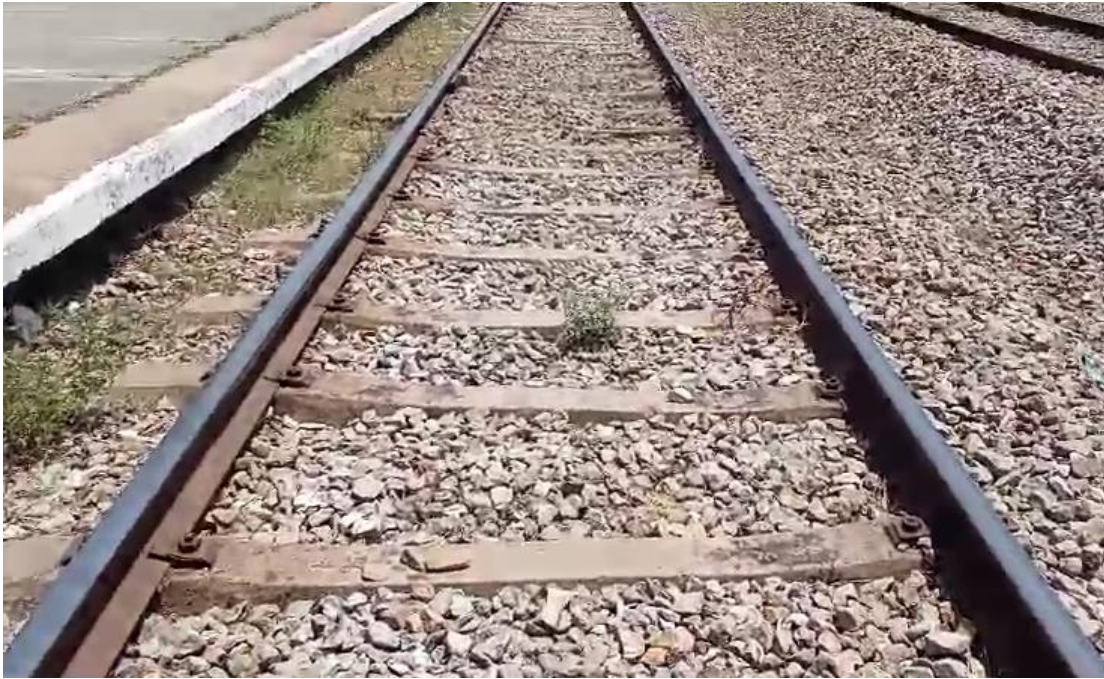
Figure 3: A Railway Track (Rawalpindi).
