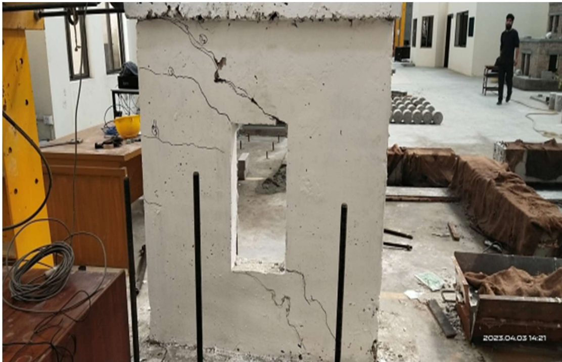
Figure 3. 6: Crack Pattern of tested wall
