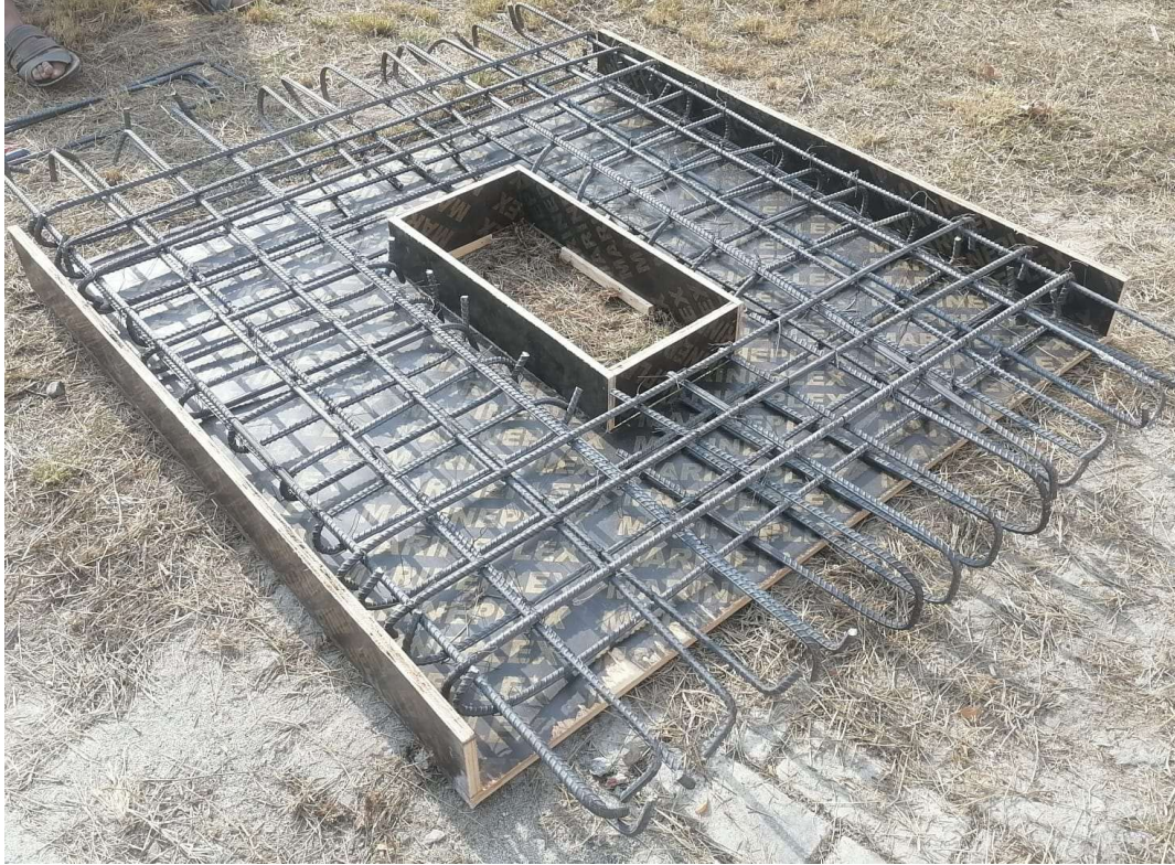
Figure 3. 2: Reinforcement of Wall web
