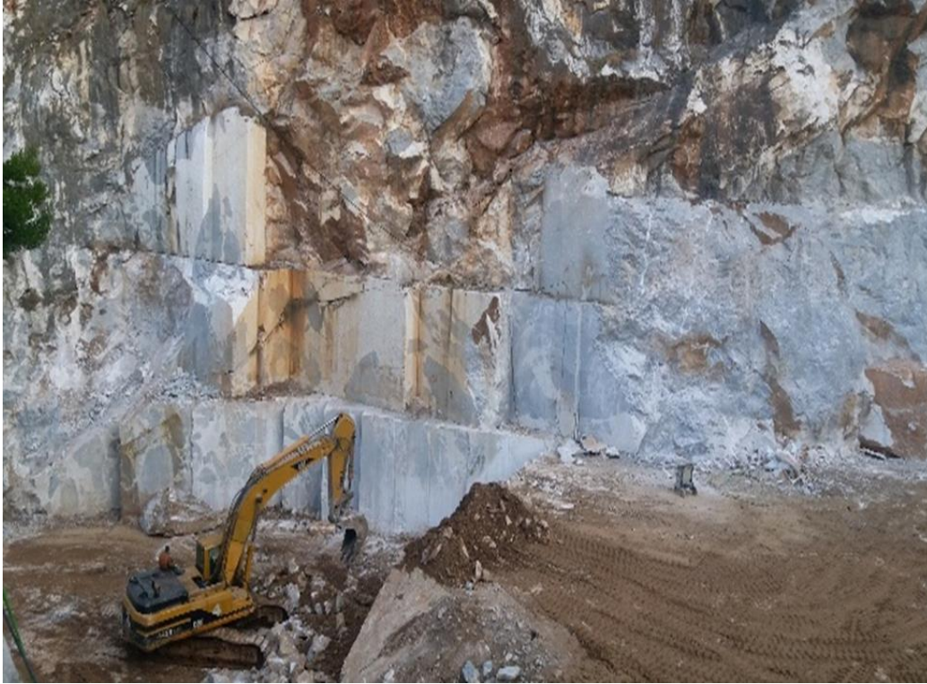
Figure 2-4: Mechanized Marble Extraction
