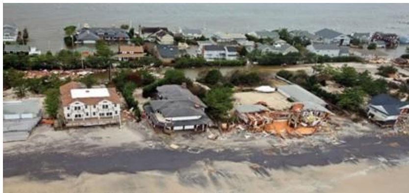
Figure 2.3.1: Coastal flood damage caused by Hurricane Sandy (Real Climate., 2014)
