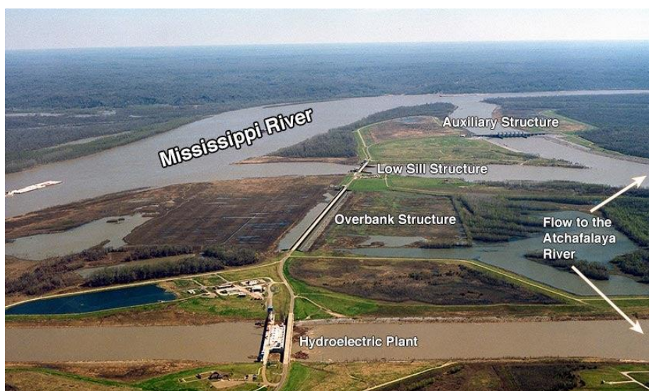
Figure 4.2.2: Aerial view of the four structures of the Mississippi River Old River Control Structure, looking downstream to the south. Water flows from the Mississippi River through the four structures, to the Atchafalaya River (right). Image credit: U.S. Army Corp
