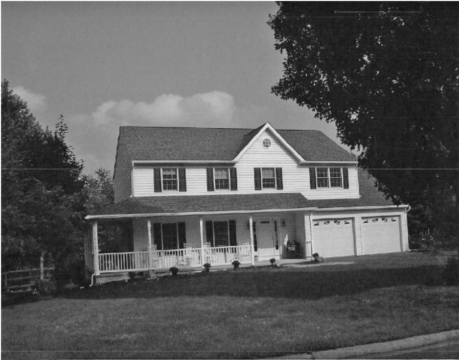
FIGURE 7.7 Photograph of the finished remodel.
