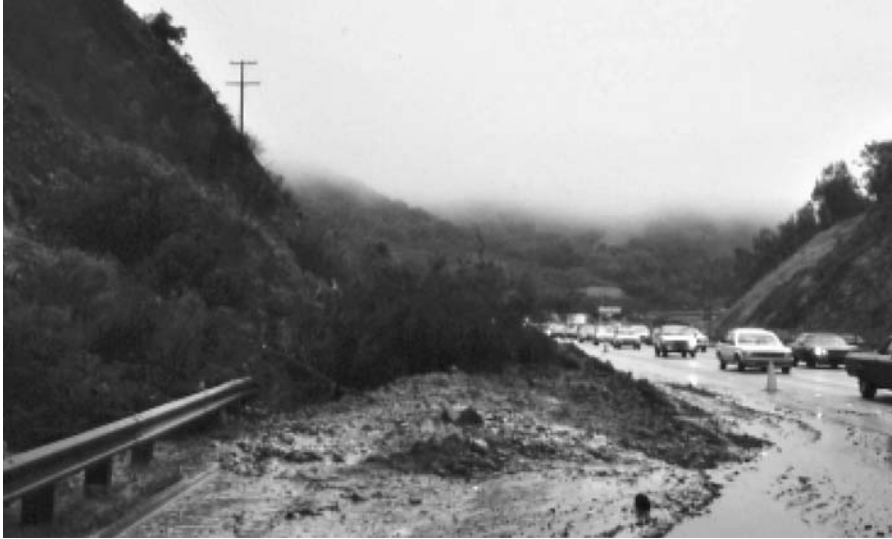
Figure 2.2 Flow slide on Highway 24 near Orinda, California. (J. M. Duncan photo.)
