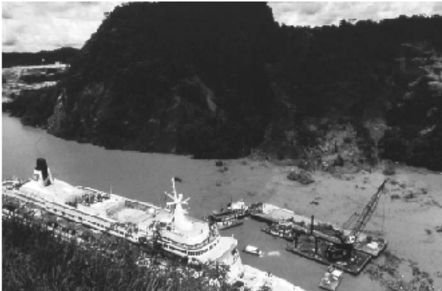
Figure 2.8 1986 Cucaracha landslide at the Panama Canal.
