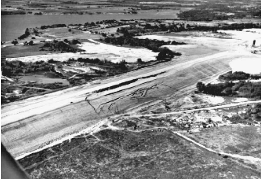
Figure 1.1 Slide in the downstream slope of the Waco Dam embankment.
