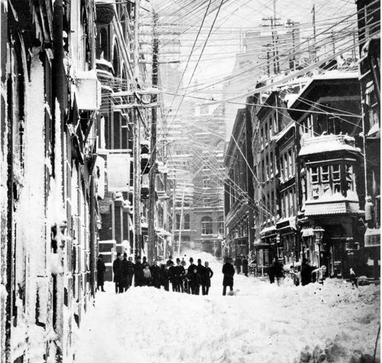
FIG 3 New York City during the Great Blizzard of 1888. The wires are a mix of telephone, telegraph, and electricity lines. ( Reproduced with permission from the Museum of the City of New York )
