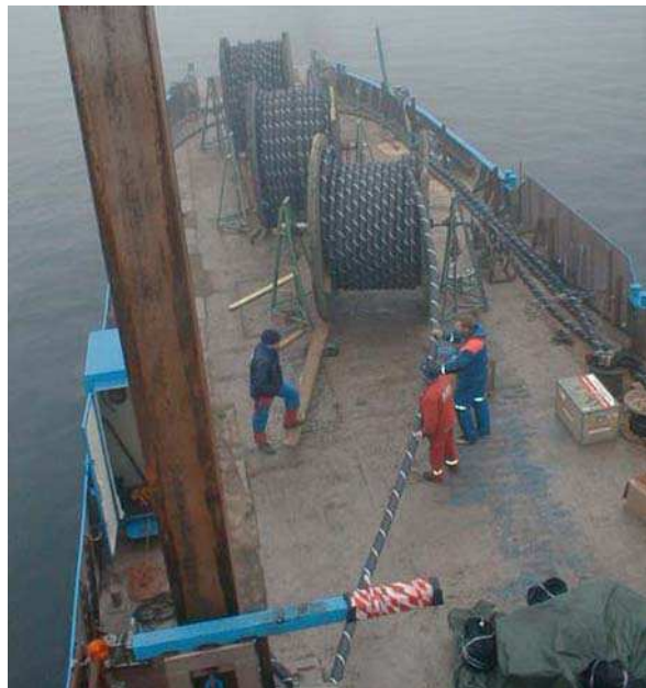
Fig. 7.7 Laying with cable drums on a barge
