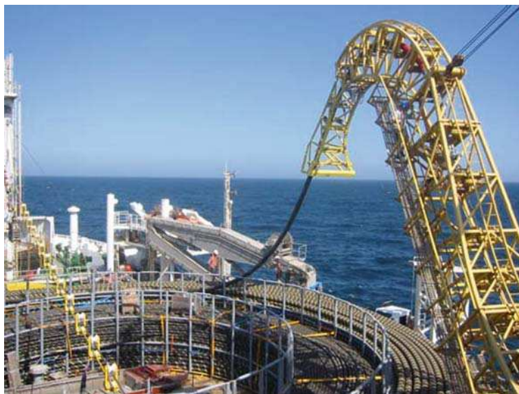
Fig. 7.6 Turntable with inner and outer partition for simultaneous laying of two cables. Here, a submarine power cable (outer partition) and a fibre-optic cable (inner partition) are stored on the turntable (Courtesy of ABB, Sweden)
