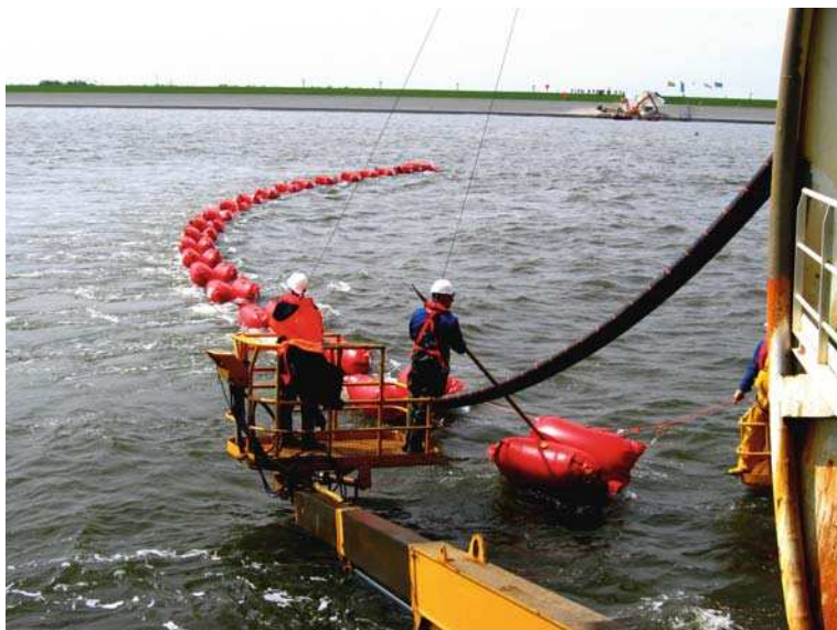
Fig. 7.15 Floating of a submarine power cable during landing (NorNed). Crew members wear safety harness
