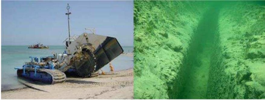
Fig. 7.26 Wheel cutter for rocky seafloor. Cable trench cut into calcarite seafloor (Courtesy of LD Travocean, France)
