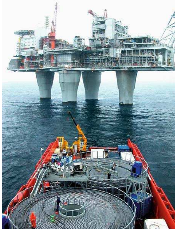
Fig. 1.3 The Norwegian gas platform “Troll A” receives its electric power supply from a pair of HVDC cables (Courtesy of ABB, Sweden)
