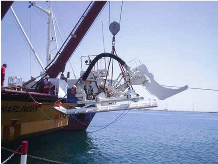
Fig. 7.25 Cable jetting device. The sword carrying water nozzles is visible to the right , tilted up (Courtesy of LD Travocean, France)
