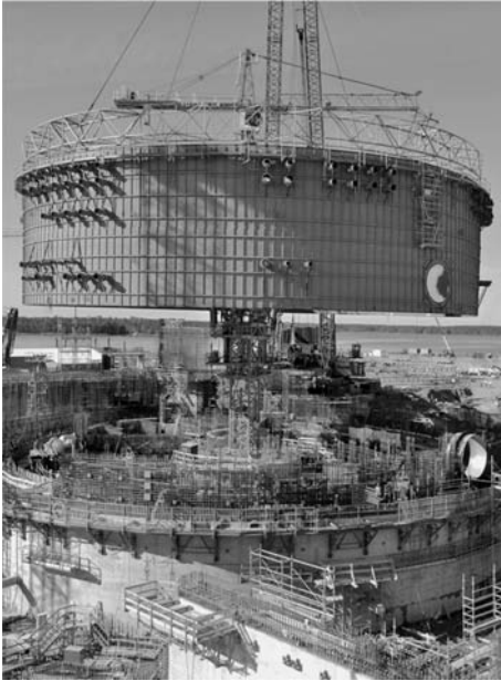
Fig. 4.20 OL3, lifting in the liner ring [22]
