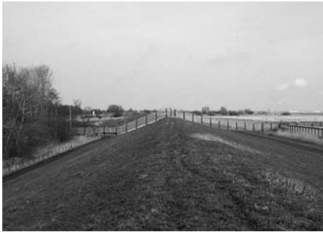
Fig. 4.7 Sea dyke as flood protection structure
