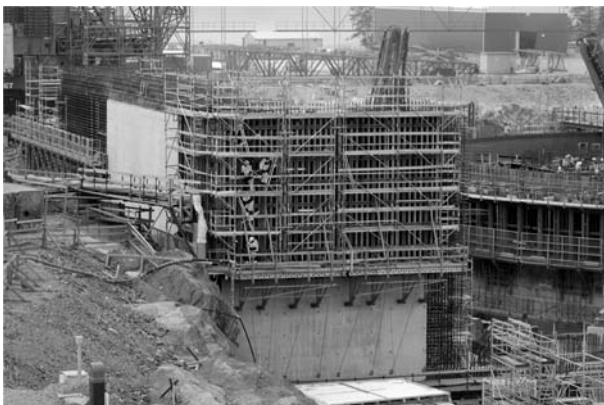
Fig. 4.18 OL3, UFA building, using large-format wall girder formwork sections [22]
