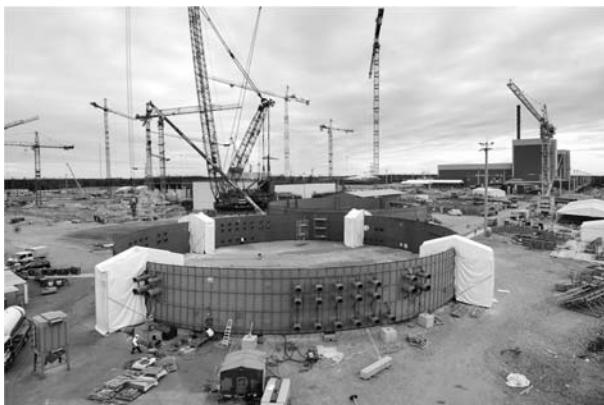
Fig. 4.19 OL3, Assembling the steel liner on site [22]
