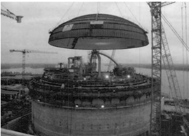
Fig. 4.21 OL3, lifting in the liner dome [30]
