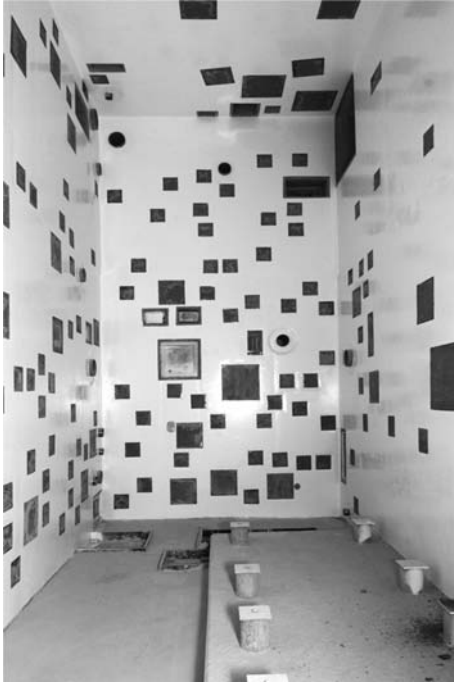
Fig. 4.23 OL3, Wall view with embedded parts in the UFA building [22]
