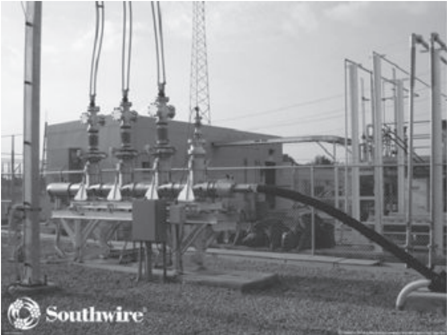
Figure 9.17 Low-voltage ULTERA cable installation in Columbus, Ohio
