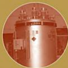
Fault Current Limiter
