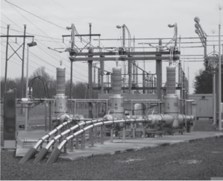
Figure 9.15 AMSC/Nexans's high-voltage cable installation on Long Island, New York
