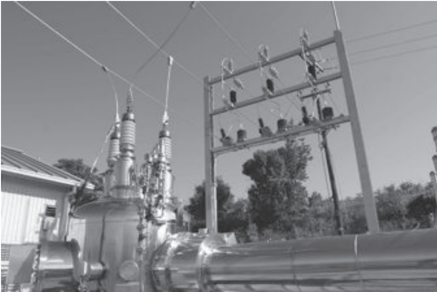
Figure 9.16 Medium-voltage SuperPower/Sumitomo's cable installation in Albany, New York
