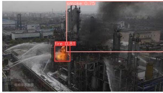
(c) Fire and smoke detected in Industry
