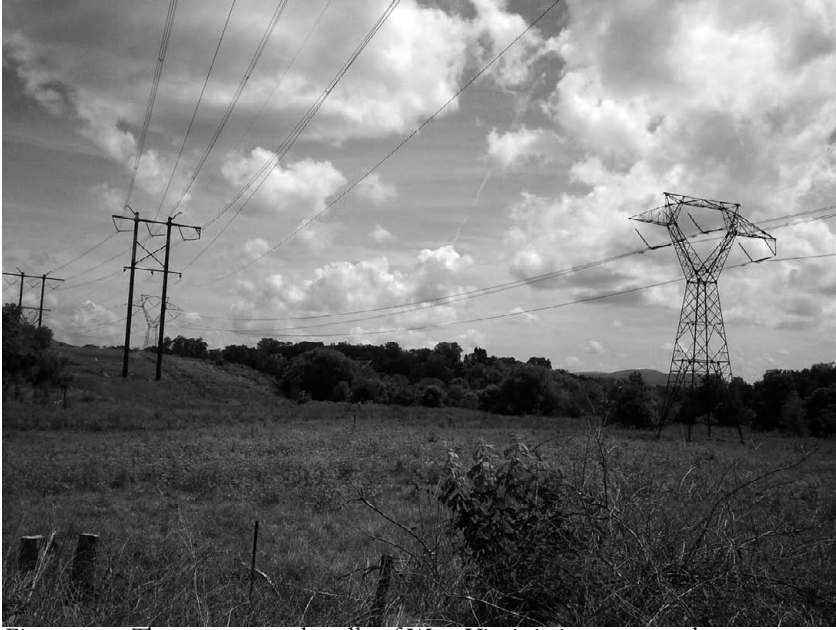
Figure 4–1. The eastern panhandle of West Virginia is cut across by transmission lines. Often, they parallel each other since transmission builders find it easier to acquire right-of-ways next to existing transmission lines or to use existing right-of-ways.
