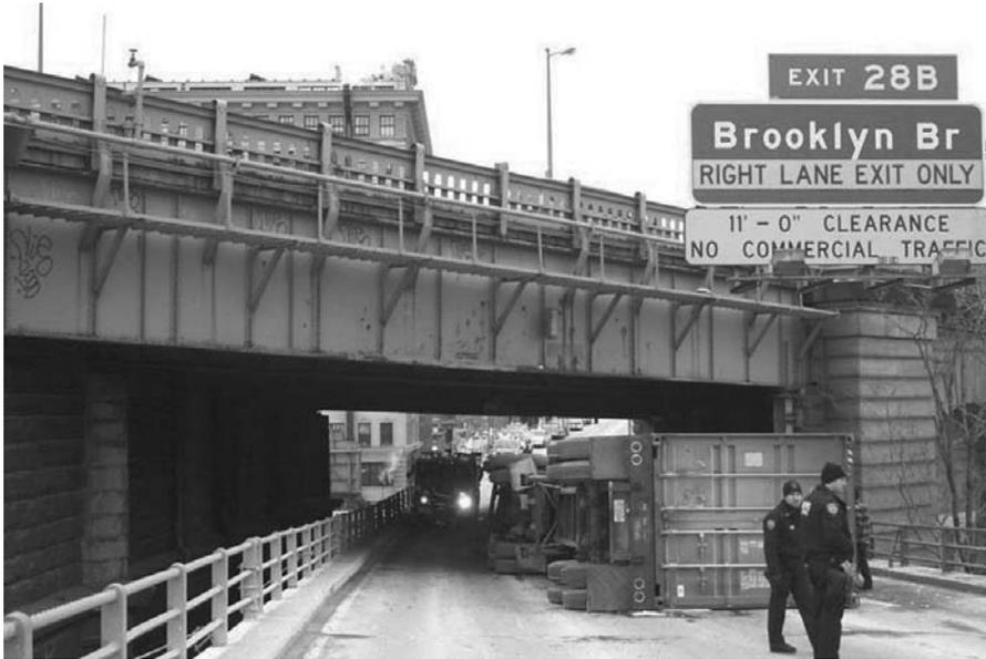
**Figure 7.1** Low overpass. Oversized overturned truck on the BQE under the Brooklyn Bridge. Photo: B. Yanev, NYC DOT.
