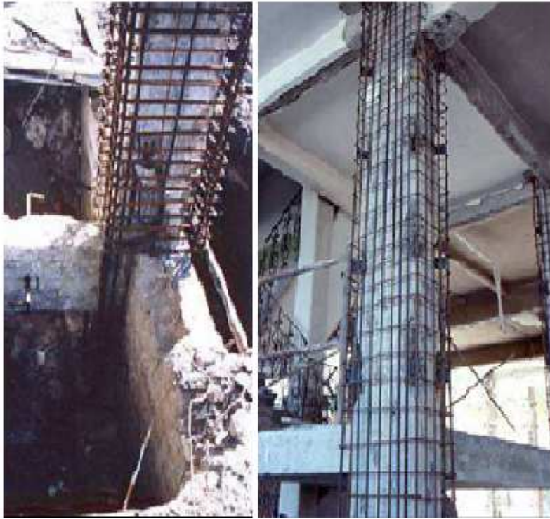
Fig 3.7: Reinforcement for Concrete Jacketing
