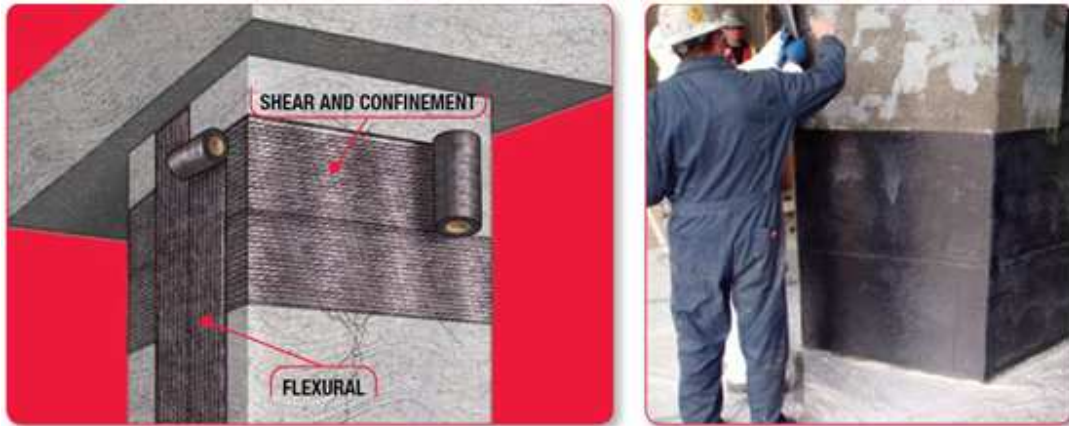
Fig 6.9: Retrofitting of column by Carbon fibers in shear ,confinement & Flexure
