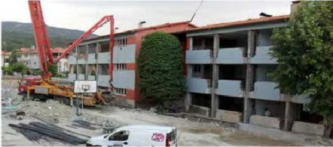
Fig 3.4: An RC jacketing application (Photo by Ahmet Sarism)
