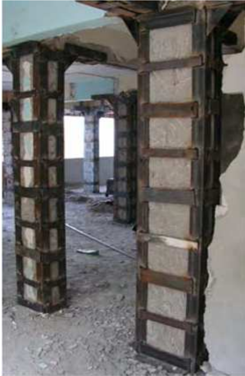
Fig 4.1: steel jacketing applied to RC columns
