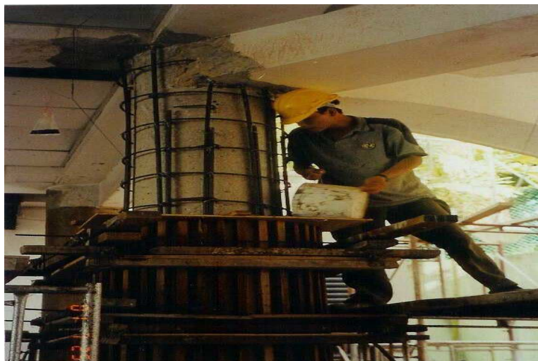
Fig. 3.1: Concrete Jacketing Is Being Applied
