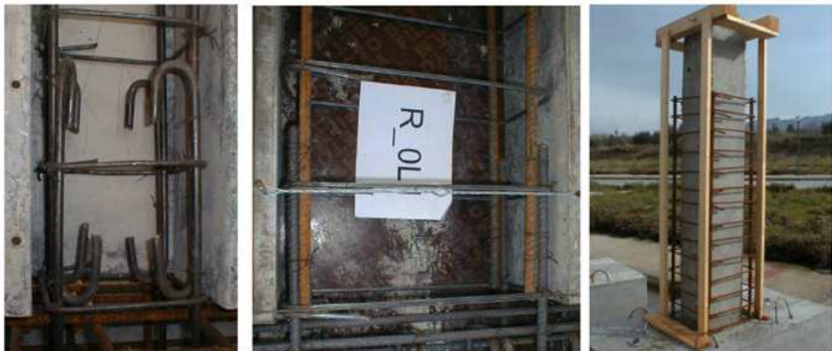
Fig 3.9: Laps at column base in type-Q specimen (left) and in type-R specimen (center); jacket reinforcement (right)
