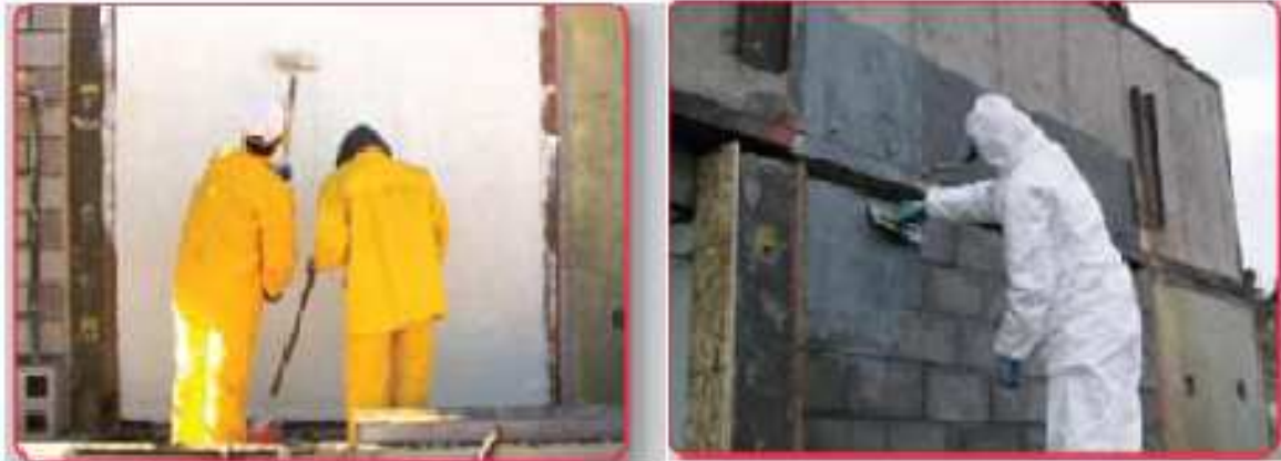
Fig 6.6: Test Walls during the construction
