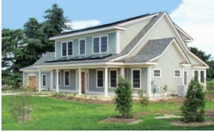
Figure 2-2 Net Zero Energy Home Residential Test Facility (NIST)
