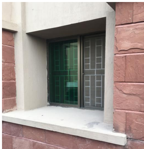
Figure 5 Window employing horizontal and vertical shading
