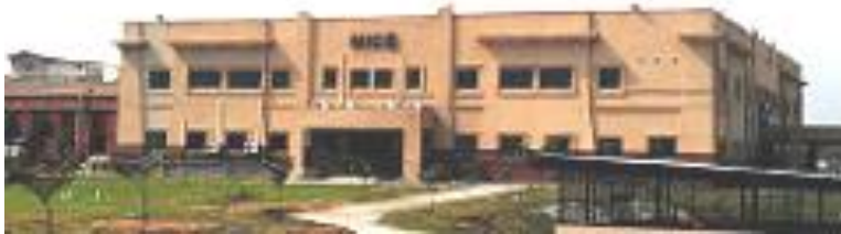
Figure 24 Main facade of NICE building
