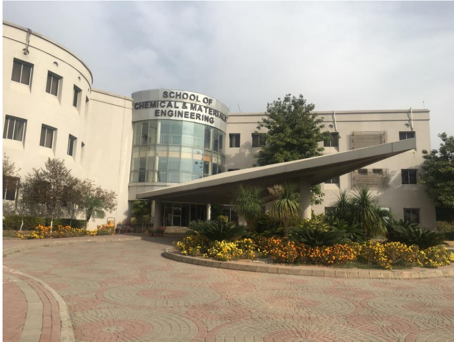
Figure 10 Main facade of SCME building
