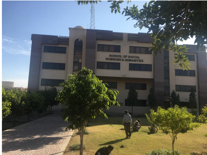
Figure 15 Main facade of S3H building
