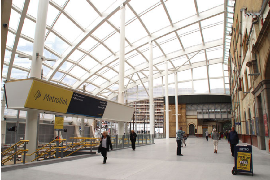
Fig. 4.2 The newly renovated Manchester Victoria Station in July 2015 ( Photo credits Chia-Lin Chen )
