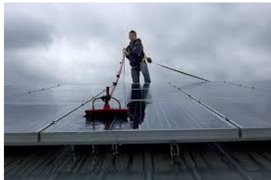
Fig. 2-19: Vacuum based cleaning [31]
