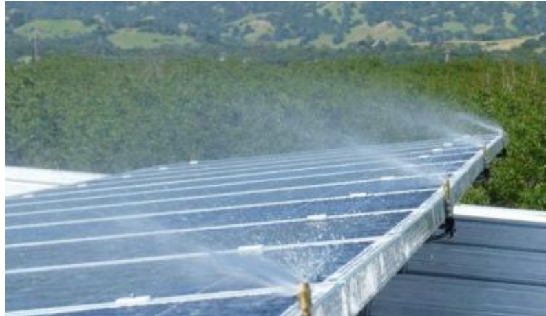
Fig. 2-20: Cleaning with water sprinklers [36]
