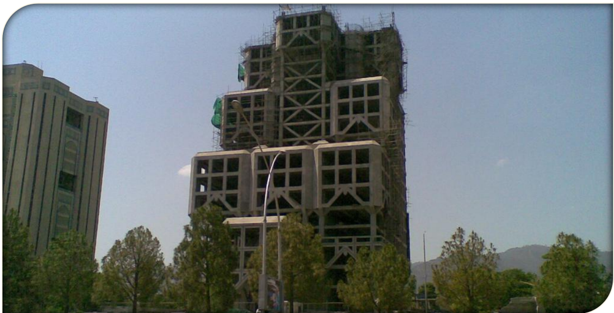
Figure 8: The State Life Building Tower, under-construction
