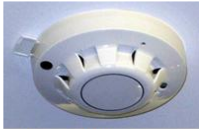
Figure 2.21: Fire sensor
