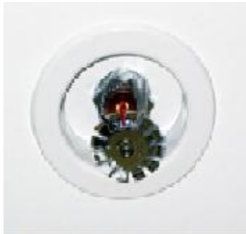
Figure 2.19: Fire sprinkler
