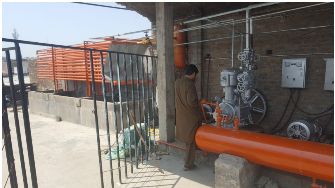
Figure1.2: Conventional Refrigeration System
