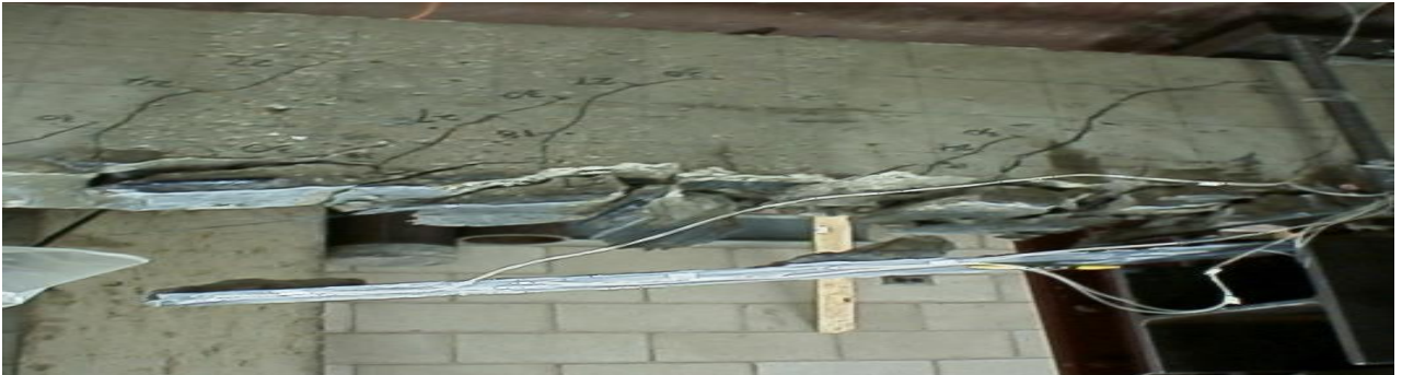
Figure 2-14: Peeling Failure of Concrete Cover
