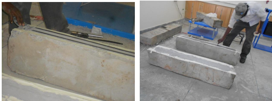
Figure 3-6: Binding CFRP to Beam using Epoxy
