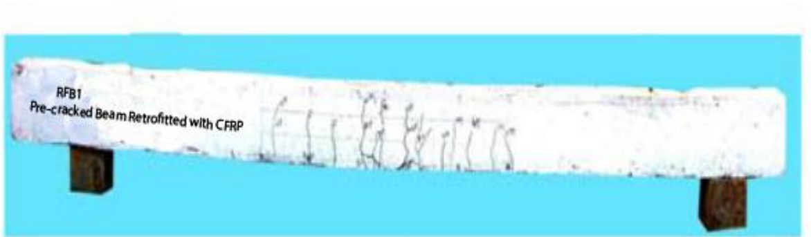
Figure 4-2: Cracking Pattern of Pre-Cracked Beam.
