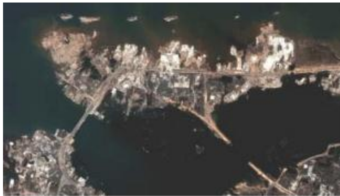
Figure 1.2 Damaged Coastlines and Bridge
