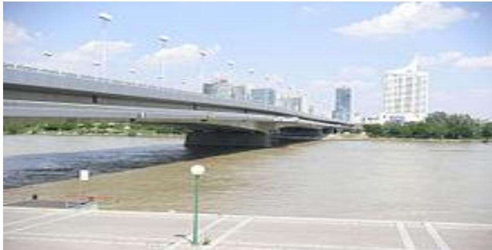
Figure 3.1 Reichsbrücke in Vienna, Austria: The rollers at the pinned bases are visible in this two-hinged arch.
