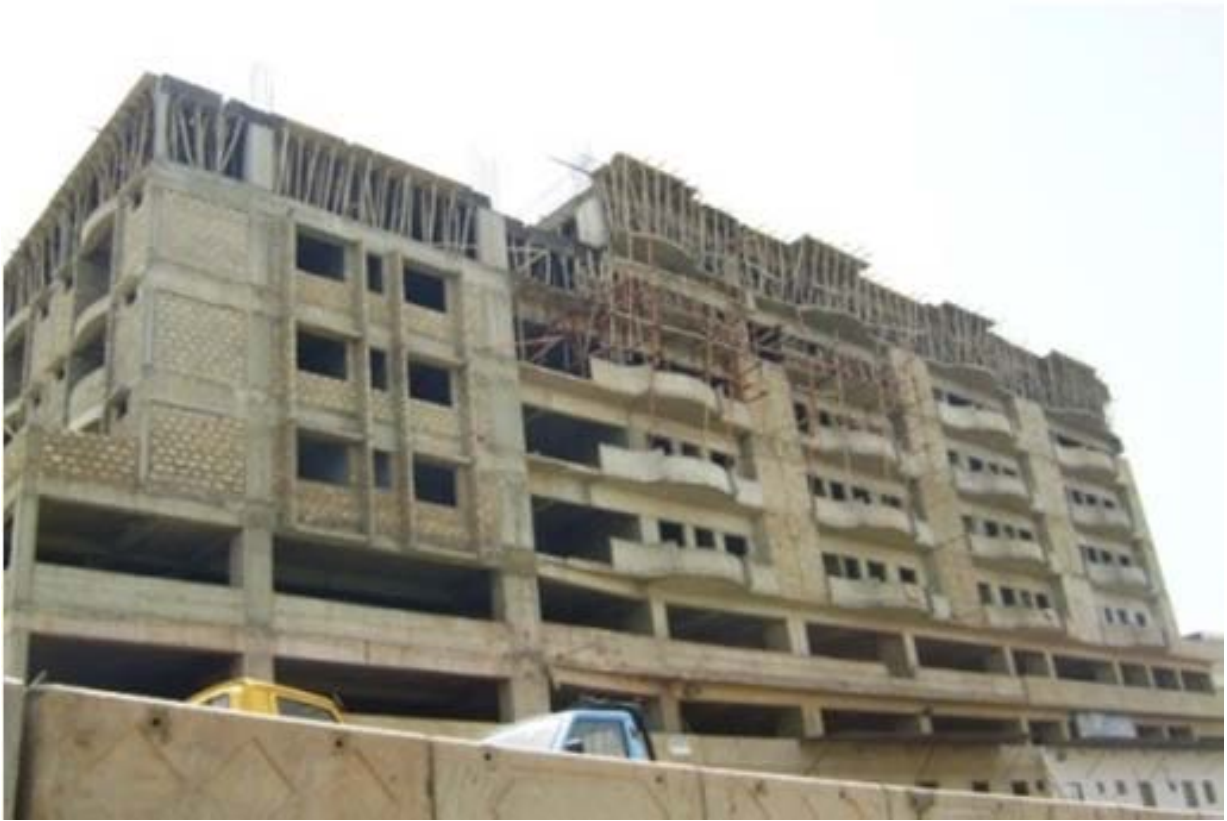
Figure 3.5: Reinforced Concrete frame structure with masonry infill in Karachi, from Lodi, (2013)
