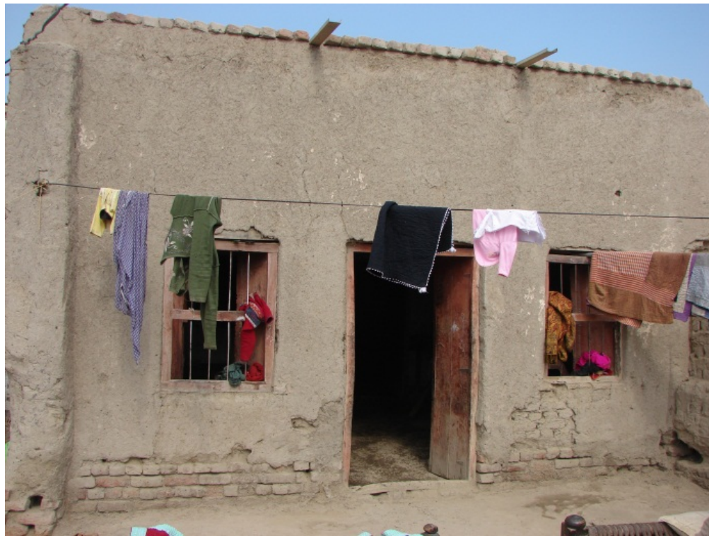
Figure 3.1: Typical Adobe construction in Pakistan, reproduced from World Housing Encyclopedia.
