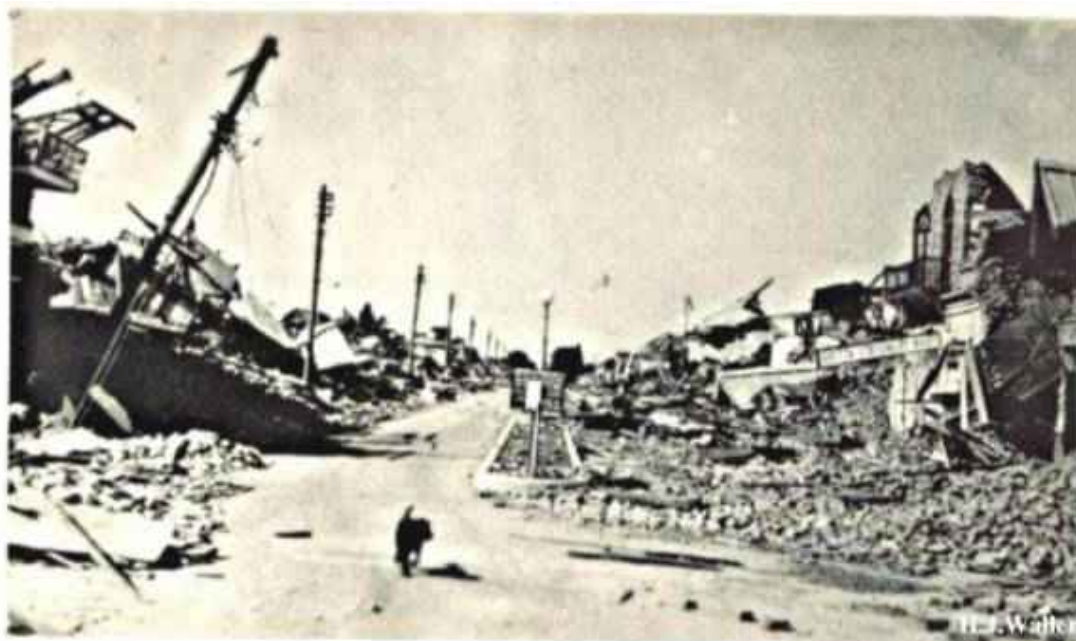
Figure 1.2: Bruce Road, Quetta. Devastation after the 1935 Earthquake
