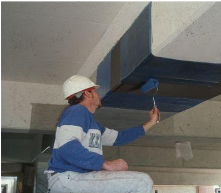
FIGURE 8-5 WORKER APPLYING FRP BELT
