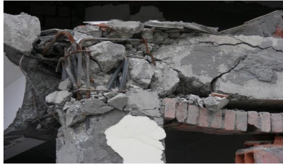
FIGURE 5-14 JOINT FAILURE
