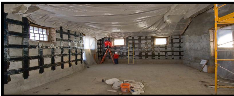
FIGURE 5-13 CFRP RETROFIT ON PARTITION WALL
