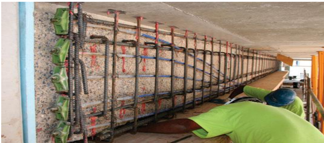
FIGURE 5-3 EXTERNAL PLATE TENSIONING
