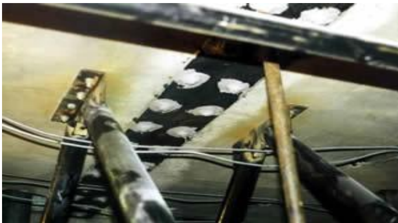
FIGURE 5-2 EXTERNAL PLATE BONDING
