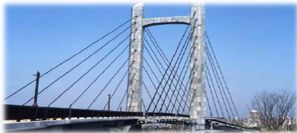
Figure 2-1:Shin-Kiba Ohashi Bridge [5]
