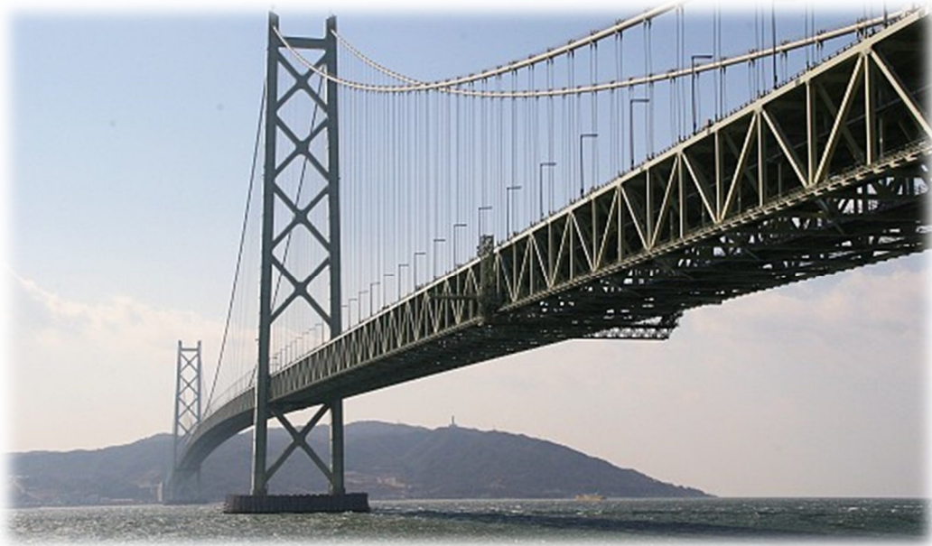
Figure 2.2: Akashi Kaikyo Bridge
