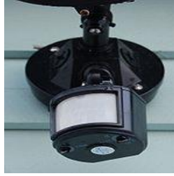
Figure 3-1: PIR motion detector used to control an outdoor, automatic light.[15]
