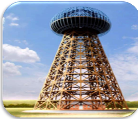
Figure 3: Wireless Transmission Tower
