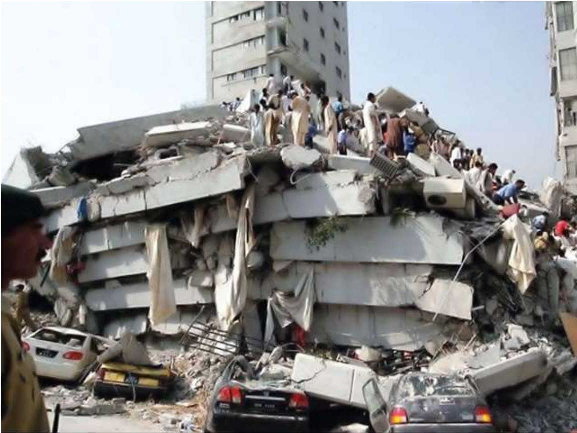
Figure 1 – Collapse of Margalla Towers
