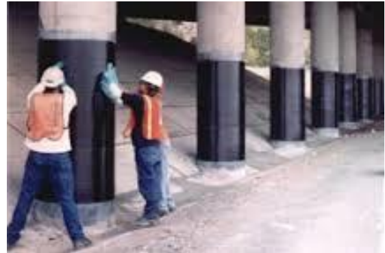
Figure 2. 5 Installation of FRP wraps on square and circular columns (Bank, 2006)
