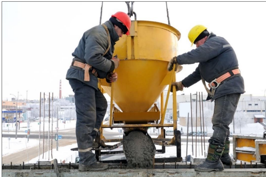
Figure 4. 10 Ready Mixed Concrete Placement
