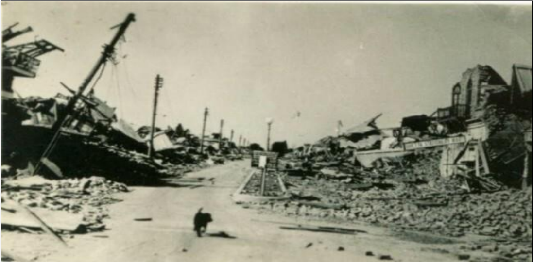
Figure 1. 3 Jinnah Road after Quetta Earthquake, 1935 (Telegraph)
