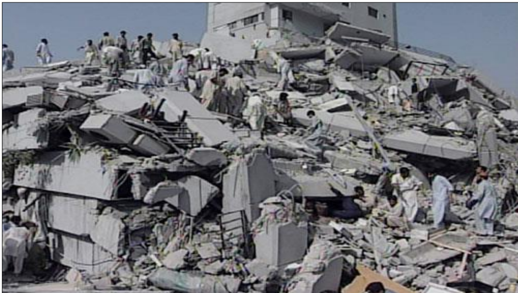
Figure 1. 4 Structural Damage of Kashmir Earthquake, 2005 ((PWP, 2011)
