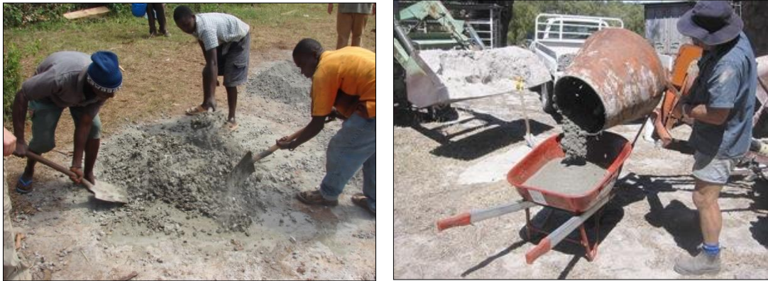
Figure 4. 9 Hand Mixing Concrete (left); Drum Mixing Concrete (right)
