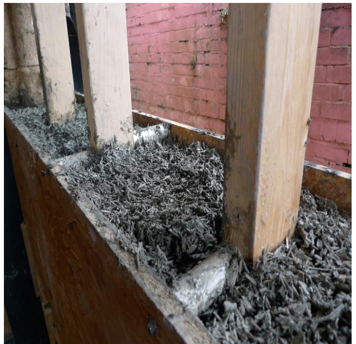
Figure 4: Application of Hempcrete
