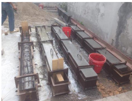
Figure 4-3: Casting of sample beams
