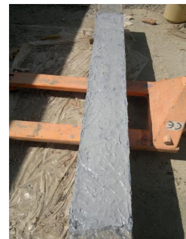
Figure 4-7: FRP wrap application
