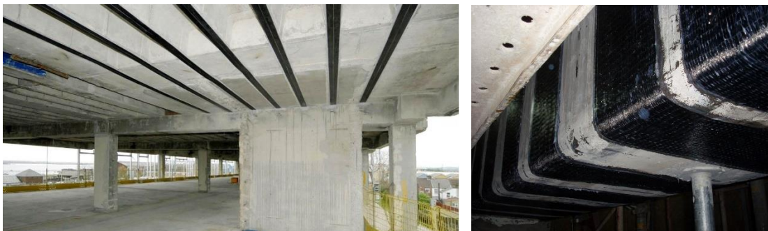
Figure 1-1: FRP retrofitting of different structures
