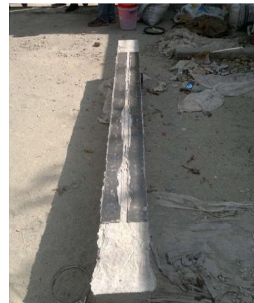
Figure 4-6: FRP double strip application
