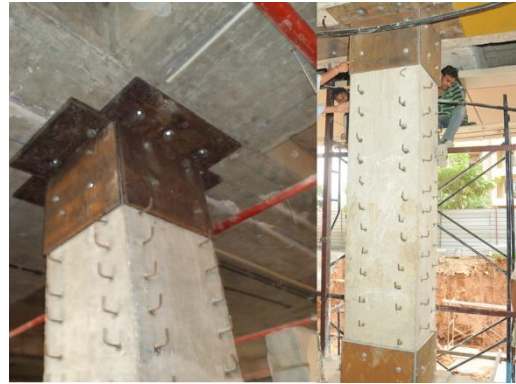
Figure 2-1: Strengthening using steel plates
