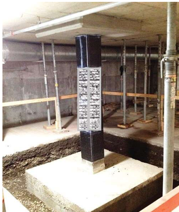
FIGURE 23 : TYPICAL COLUMN WRAP
