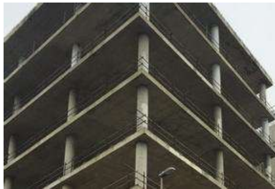
FIGURE 3 : FLAT PLATE
