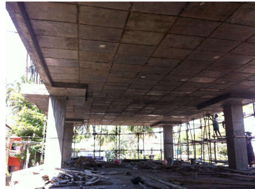
FIGURE 2 : FLAT SLAB
