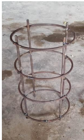
Figure 5 Reinforcement without GW Mesh
