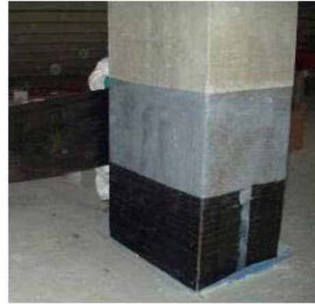
Figure 2. Application of FRP for seismic retrofitting of RC columns
