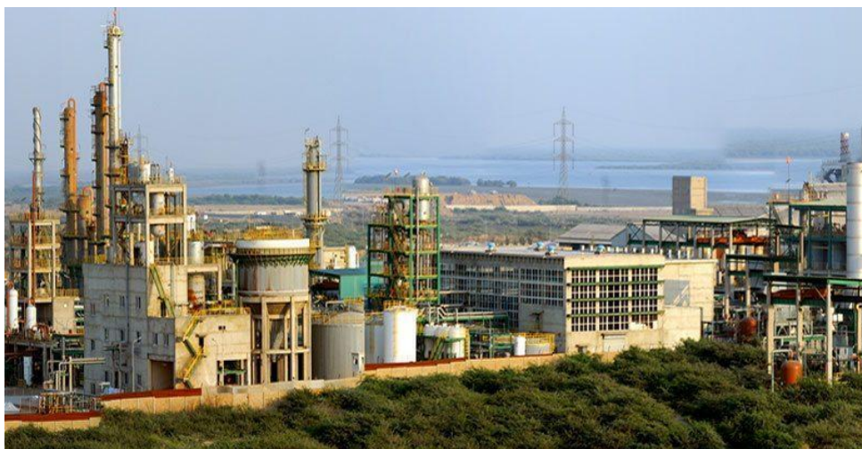
Figure 1 EPCL Karachi Plant
