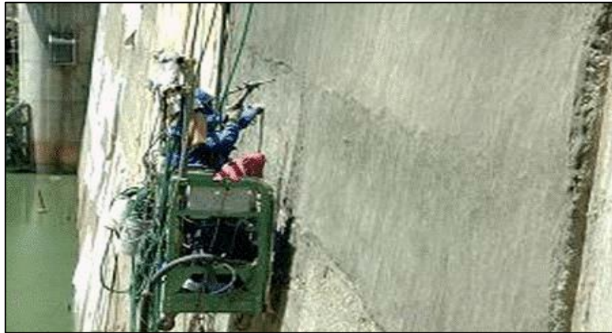
Figure 2.10: Application of ECC for repair of Mitika Dam
